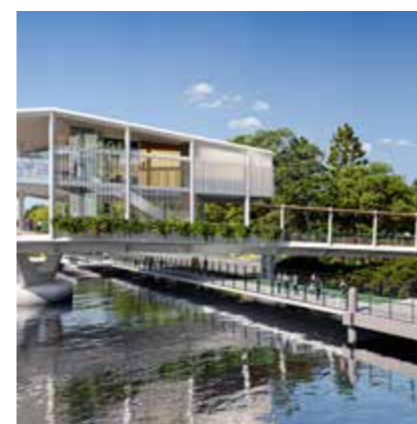
Kangaroo Point Green Bridge $190.2 Million
