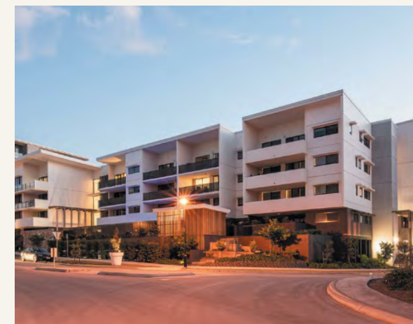
HIGH STREET - COMPLETED 2018
