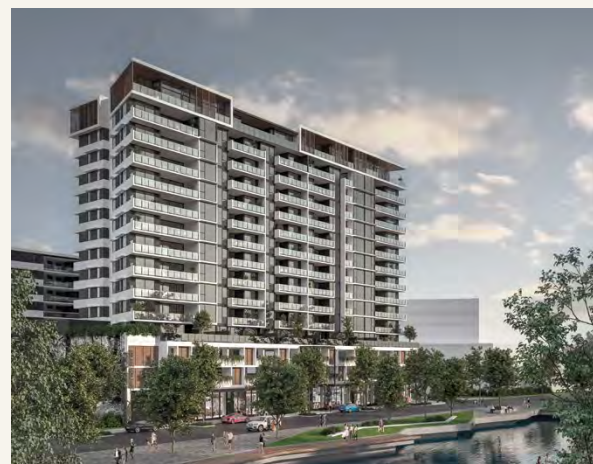
THE CORSO - UNDER CONSTRUCTION
