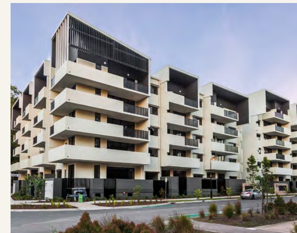
FOREST EDGE & BOTANICA - COMPLETED 2020
