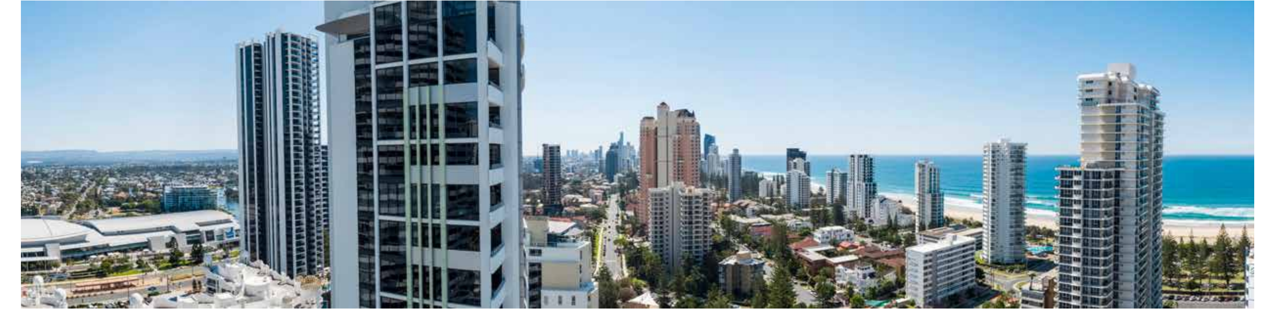
NORTH WEST – NORTH EAST
