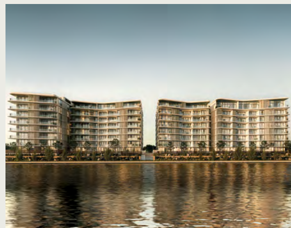
ST CLAIR - UNDER CONSTRUCTION
