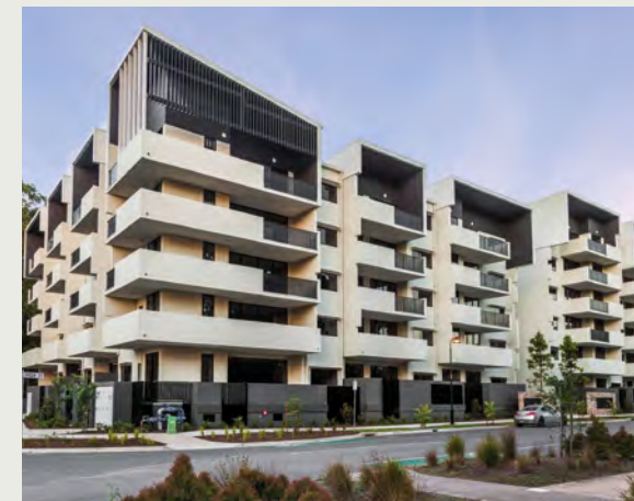
FOREST EDGE & BOTANICA - COMPLETED 2020
